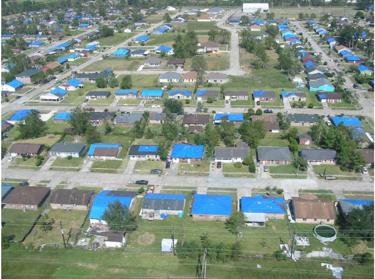
Neighborhood in Jefferson Parish, which mostly had wind damage and not flood damage.
