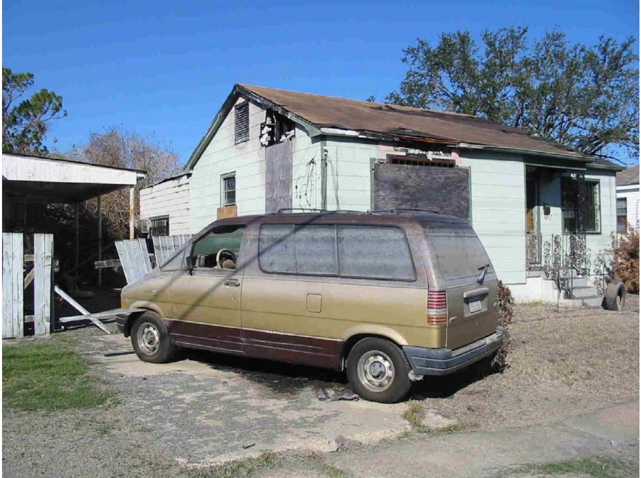
Vacant neighborhood in New Orleans. The white on the vehicle is from salt in the flood water. Notice the high water mark at the top of the vehicle.
