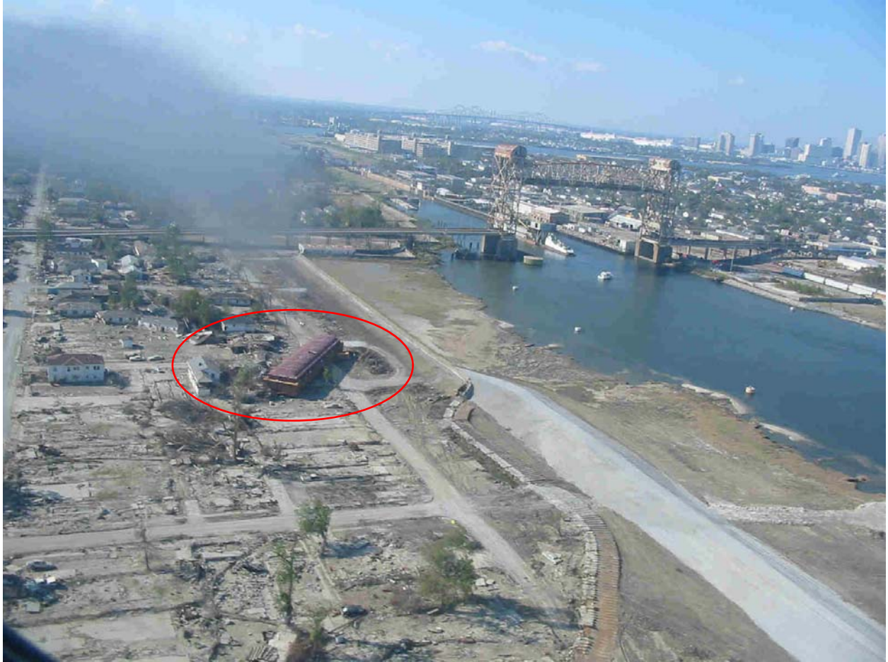
9th Ward in New Orleans near a levee breach. Notice the barge flipped over and on top of a house and school bus.
